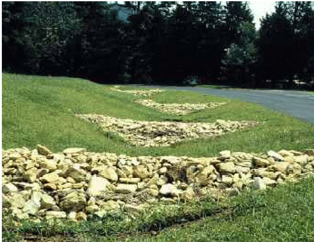
Figure 6-3 Grass Swale with Check Dams (VA DEC, 1999)
