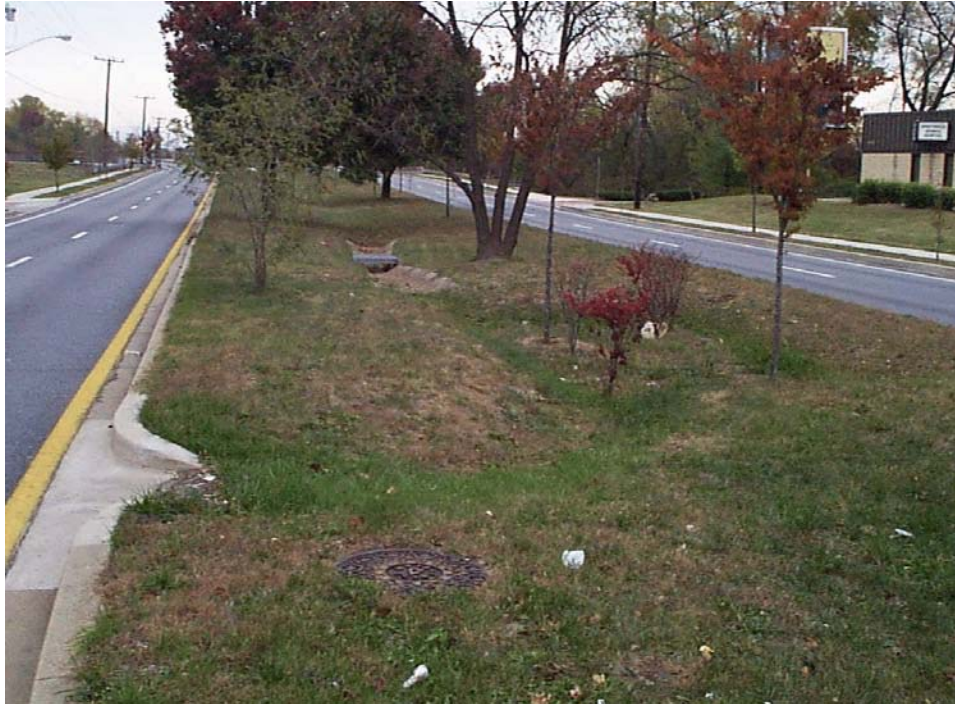
Figure 7-5 Bioretention Application in a Roadway Median
