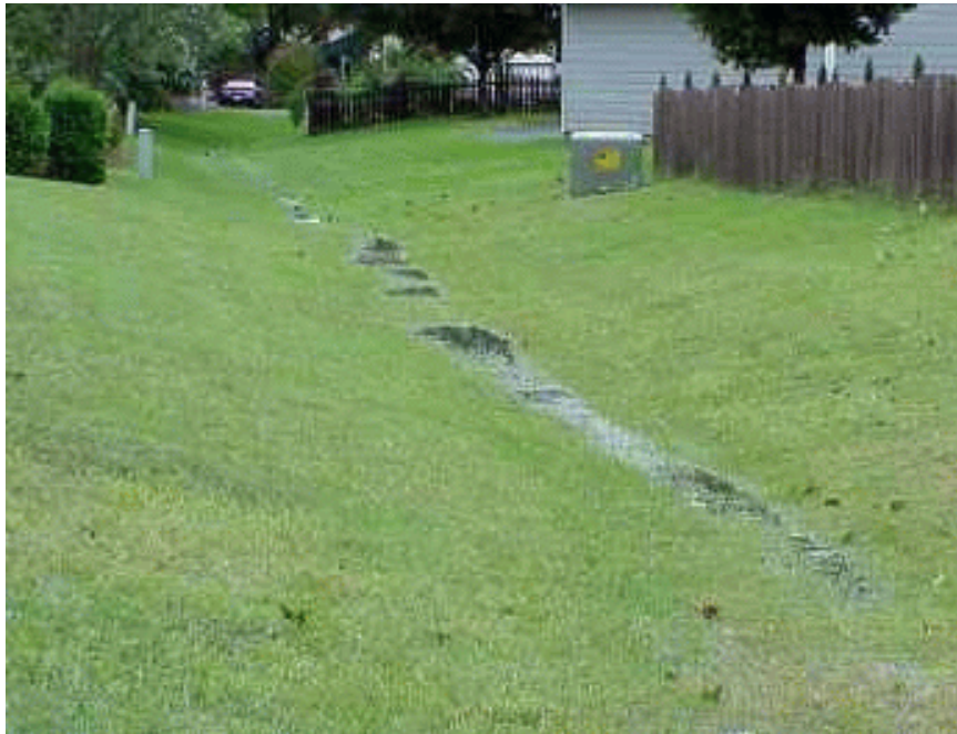
Figure 6-1 Grass Swale (VA DCR, 1999)
