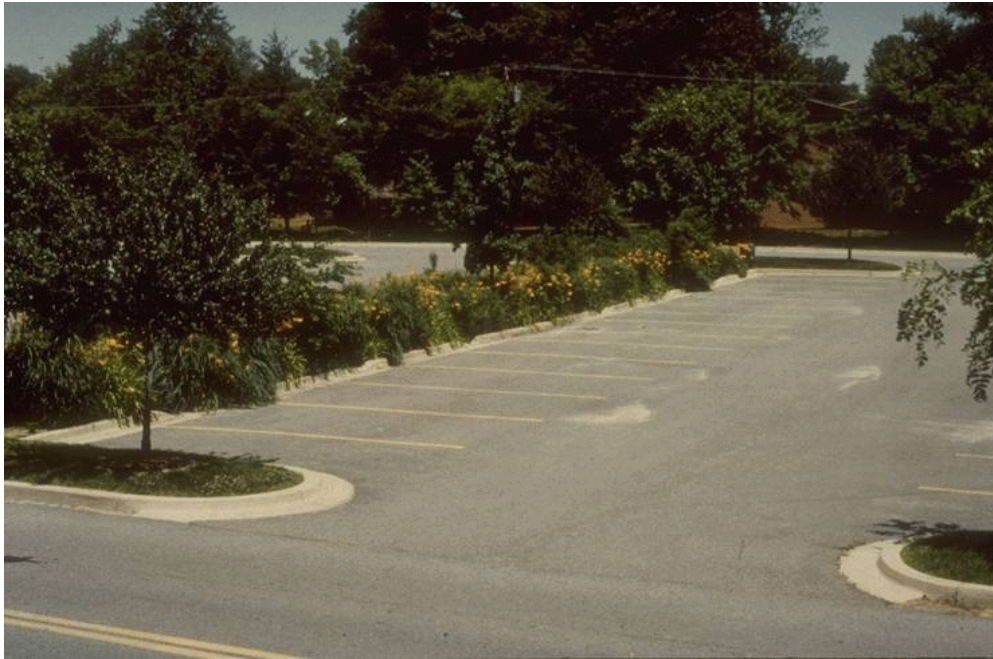
Figure 7-3 Bioretention Application on New Parking Lot
