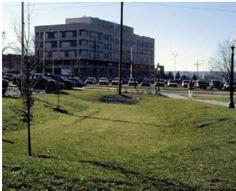
Figure 6-2 Grass Swale with Check Dam (VA DEC, 1999)
